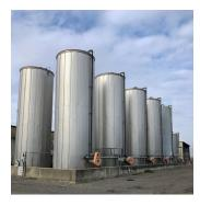
Includes tank farm with (10) 30,000 gallon vertical tanks with insulation, side entering agitators, and electrical insertion heaters. 4 for B-100, 4 for feedstock, 1 for crude glycerin, and 1 for methanol. The BN rail line is next door and BN approved a switch onto property but rail line was never built.
